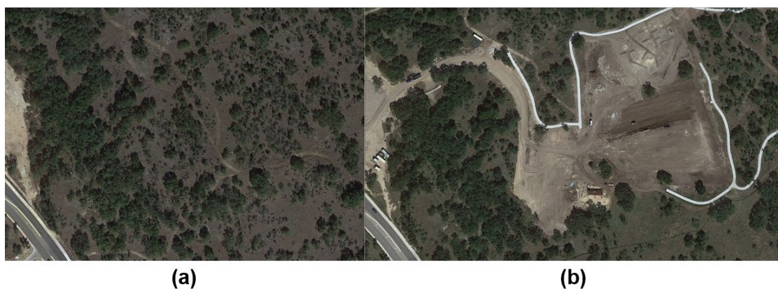
Figure 59: Google Earth® images pre- and during construction: (a) 03/01/2021 and (b) 10/29/2021
