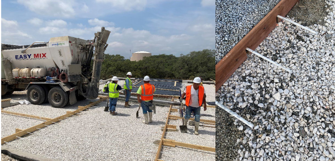
Figure 10: Construction of the PC pavement
