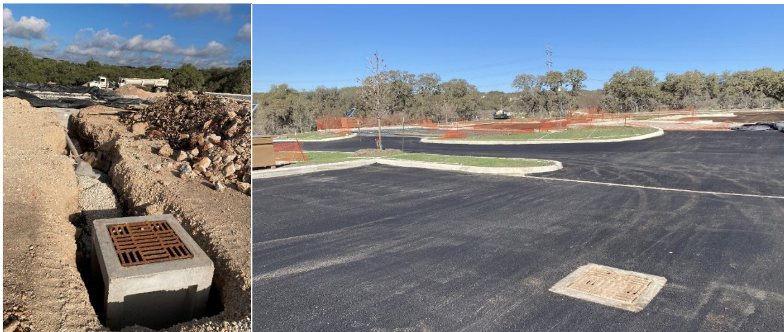
Figure 6: Surface drain for the CP (i.e., impermeable) pavement
