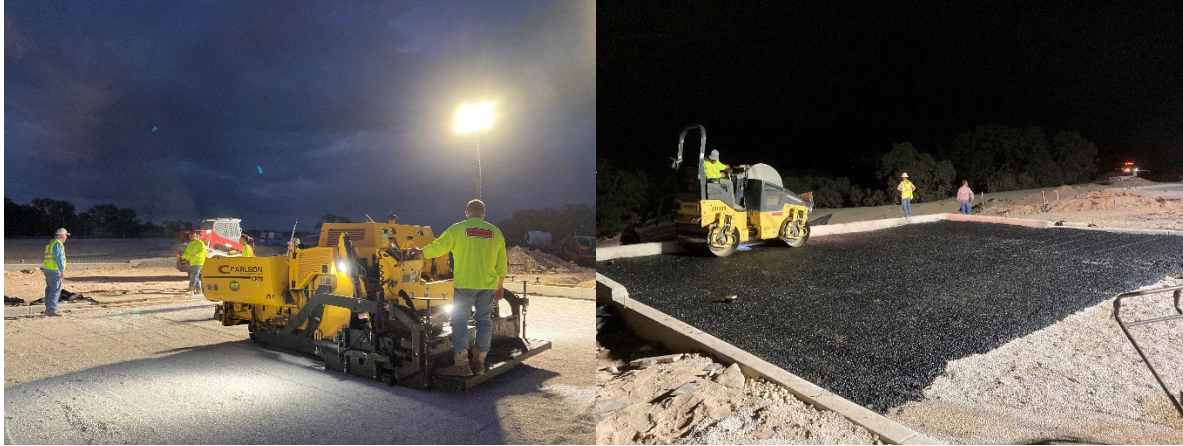
Figure 9: Construction of the PA pavement
