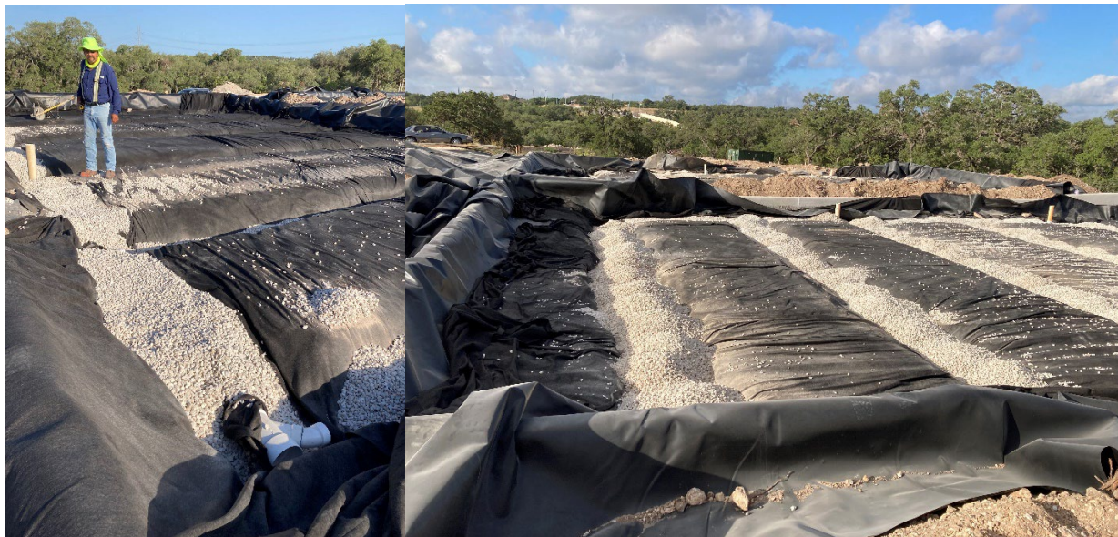
Figure 3: Construction of the liner and perforated drain lines backfilled with gravel
