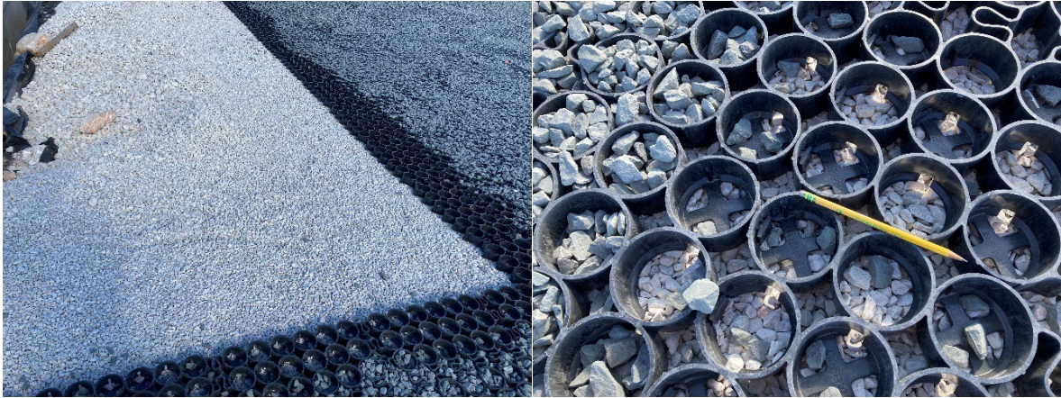
Figure 7: Construction of the PGr pavement
