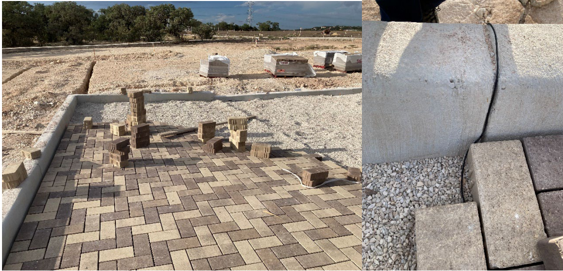
Figure 11: Construction of the PICP. Note temperature sensor lead wires.
