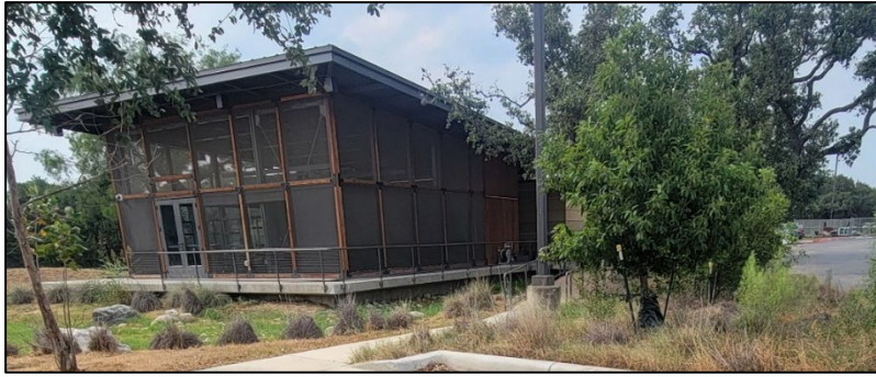
Figure 2 – The Mesquite Living Lab facility.
