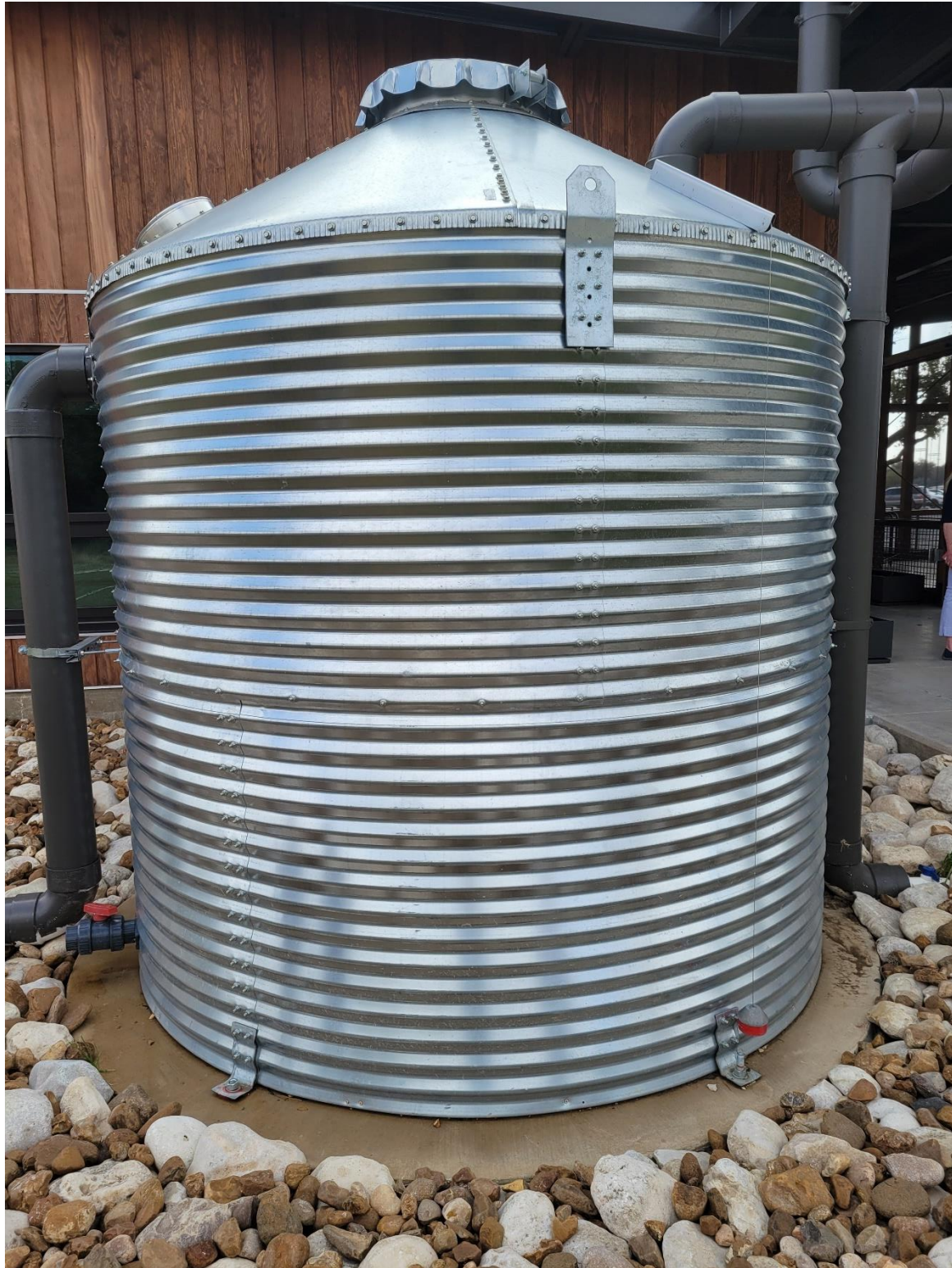
Figure 3.9. Photograph of the cistern at the Mesquite Living Laboratory.
