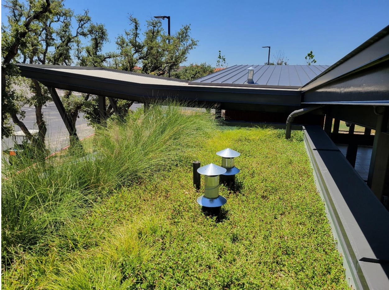
Figure 3.10. Photograph of the green roof atop the restroom facility at the Mesquite Living Laboratory.
