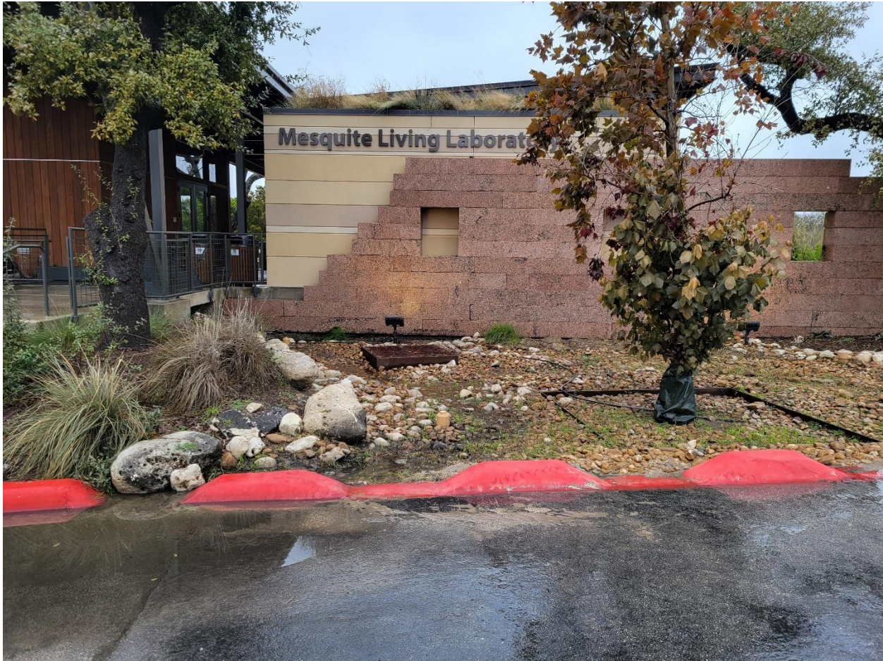
Figure 3.1. Photograph of the Mesquite Living Laboratory, showing the curb cuts that allow parking lot runoff to flow into the bioretention basin in front of the building and the repurposed pink granite forming the building façade. The sycamore tree in the foreground is planted in a tree box within the bioretention basin. The other trees in the picture are live oaks and were preserved through construction of the building. Plants on the green roof are also visible just above the building sign.
