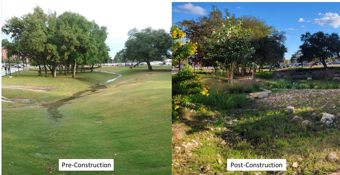
Figure 4. Before-after photos looking downstream, showing the mowed channel in the pre-construction condition and the north basin of the bioretention basin two years post-construction.
