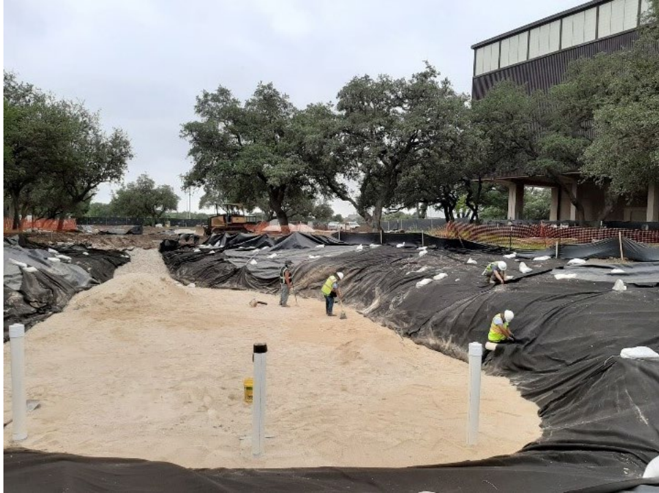
Figure 5. Photograph showing the impermeable liner and basin partially filled with sand and biomedix mix.
