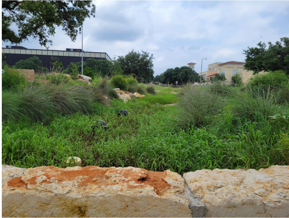
Figure 7. Photograph showing the bioswale. Picture orientation is looking upstream toward the unmowed grassy channel and bioretention basin.
