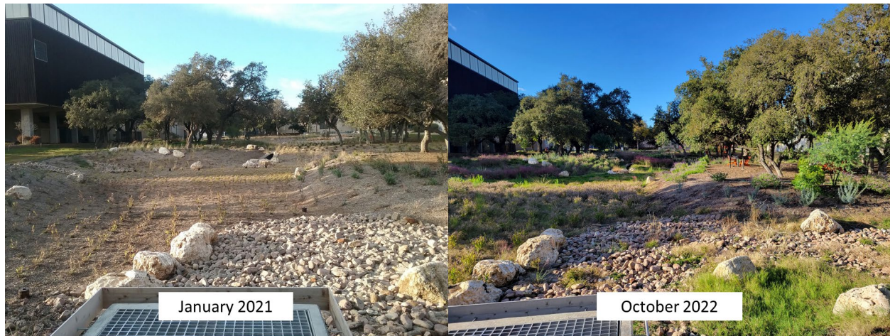
Figure 15. Photographs show growth of planted vegetation in the bioretention basin over time. The left photo was taken two months after basin construction, the right photo was taken almost two years after basin construction.
