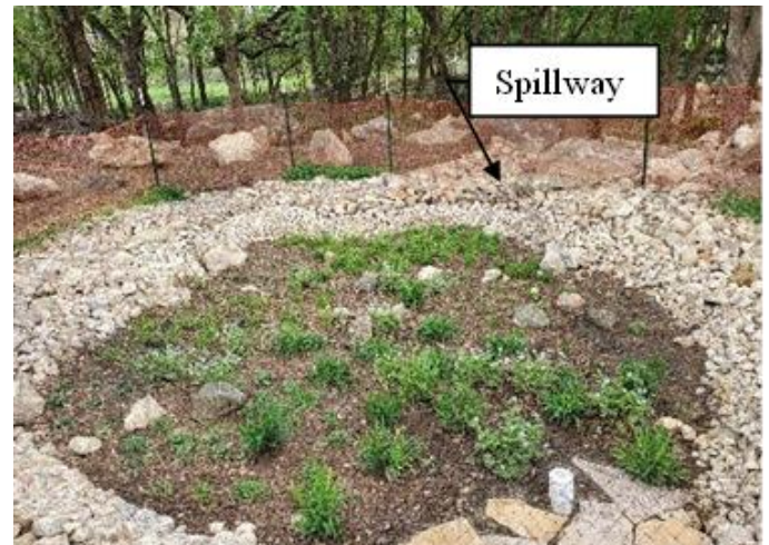
Figure 6: Completed Basin with Spillway That Overflows into the Enhanced Natural Bioretention Area
