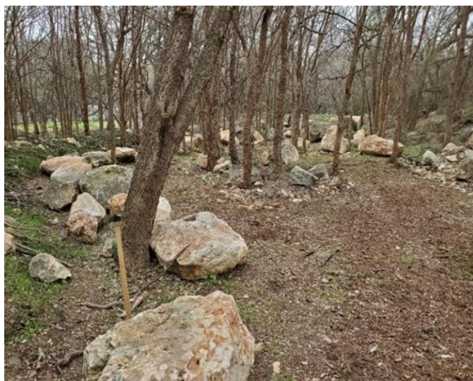
Figure 9: Berm Showing Revegetation and Placement of Boulders at Toe and Walking Path to the Right
