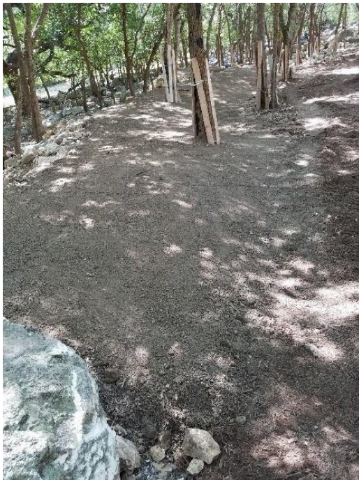
Figure 8: Completed 3:1 Berm on Northside of Area.
