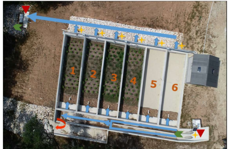
Figure 1 – Aerial view of the LID testbed, water movement and monitoring locations.
