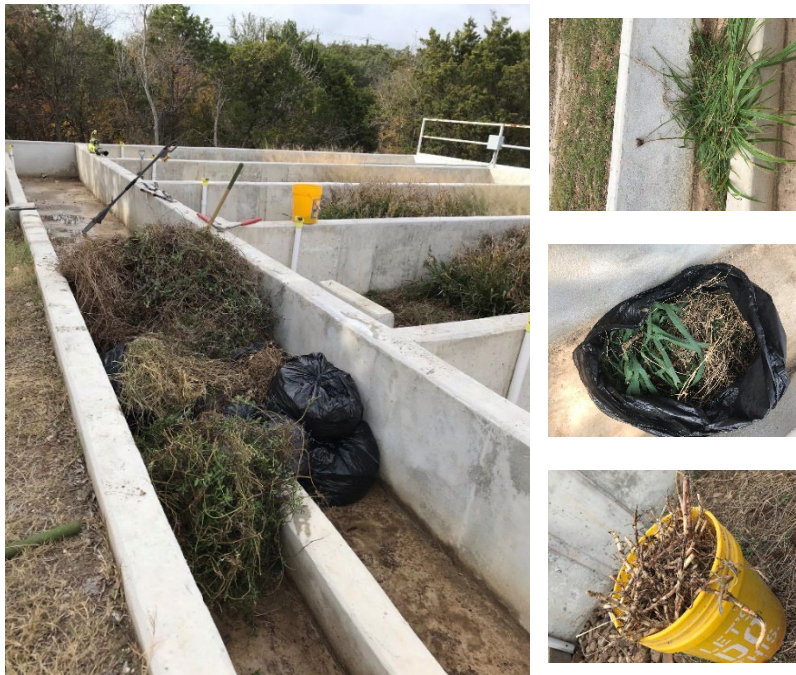
Figure 6- 1. Monthly and annual maintenance to remove debris, weeds and dead plants
