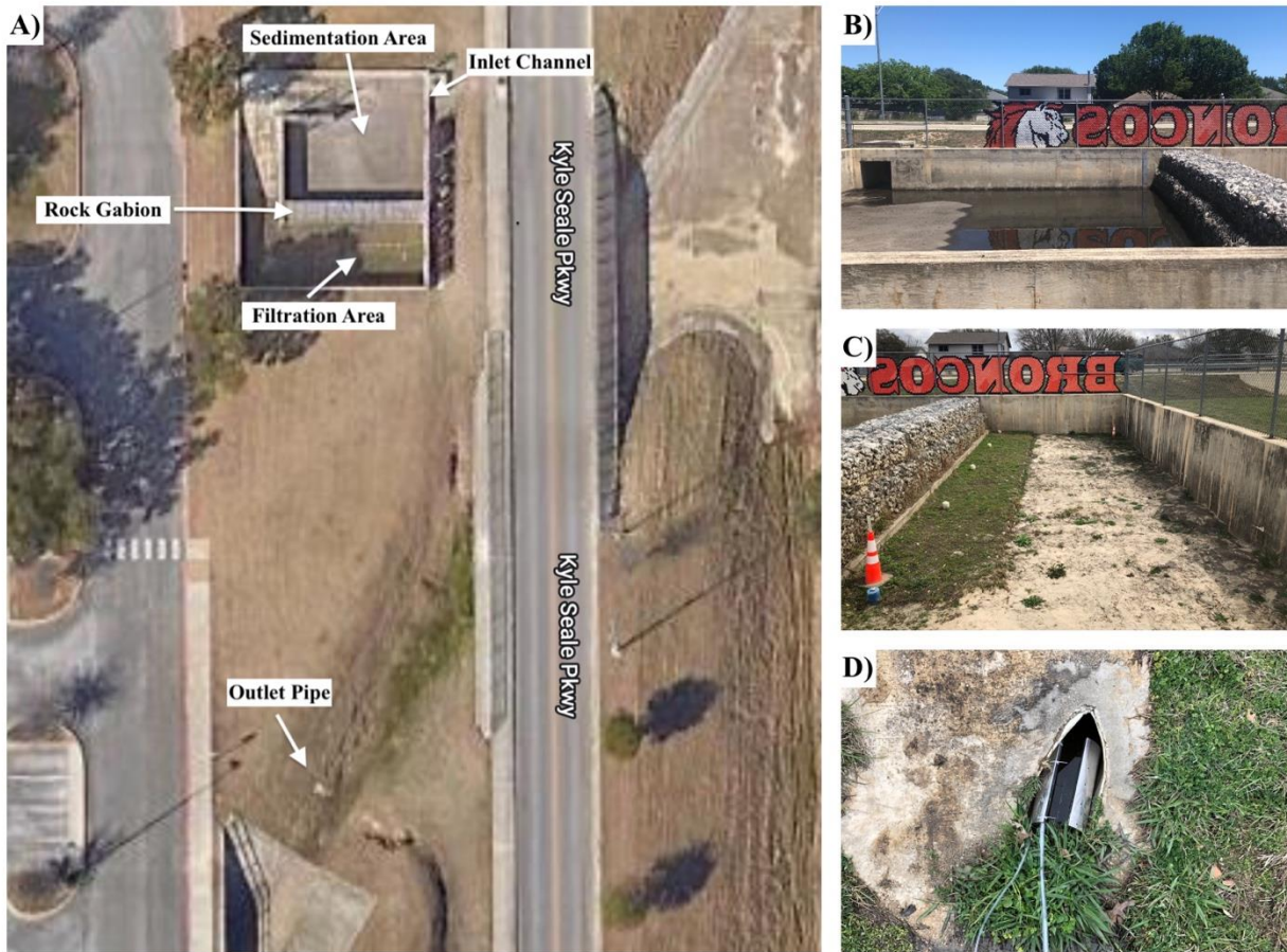
Figure 43. Kyle Basin A) plan view image of Kyle site with the inlet channel, sedimentation area, filtration area, rock gabion and outlet pipe B) sedimentation area and inlet channel C) filtration area and rock gabion D) Outlet pipe.
